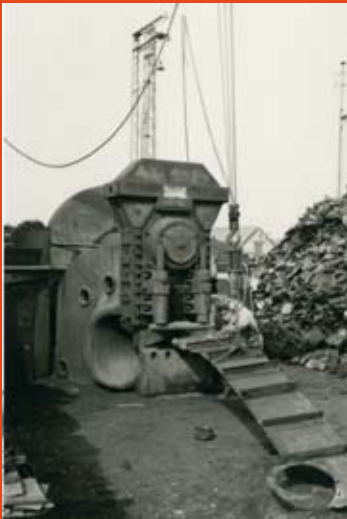
Cutting scrap around World War I with the help of mechanical guillotine shears. Photo: Frank Rijdsdijk NV, The Netherlands.
