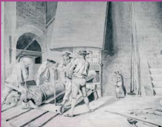
Recycling of bronze: in 1778, a cracked bronze cannon is remelted at the Royal Brass Foundry in Woolwich, England.
