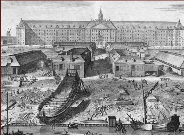
Shipbreaking in the 17th century was carried out by reversing the process of ship construction. An old engraving of a marine shipyard in Amsterdam.
